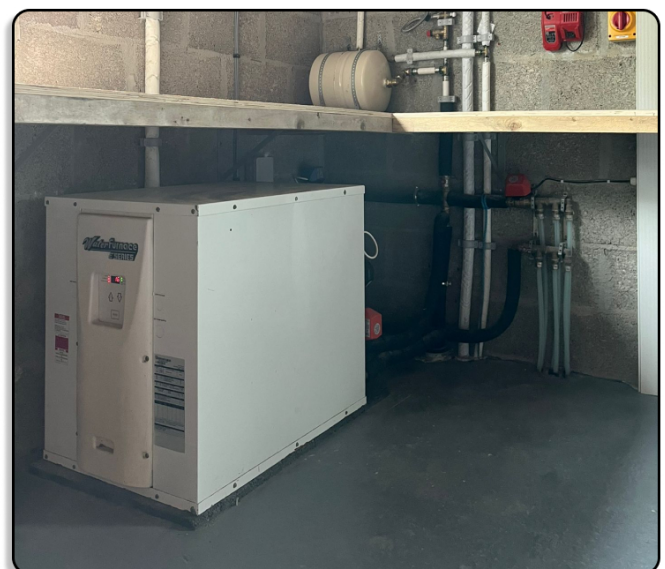
RESIDENTIAL, 8KW COOLING, X3 UNDERFLOOR ZONES & HOT WATER
