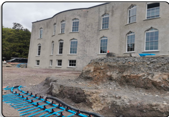
GLENGARRIFF CASTLE BRINE TO WATER (62kW) & UNDERFLOOR HEATING, CLOSED HORIZONTAL HEAT COLLECTOR
