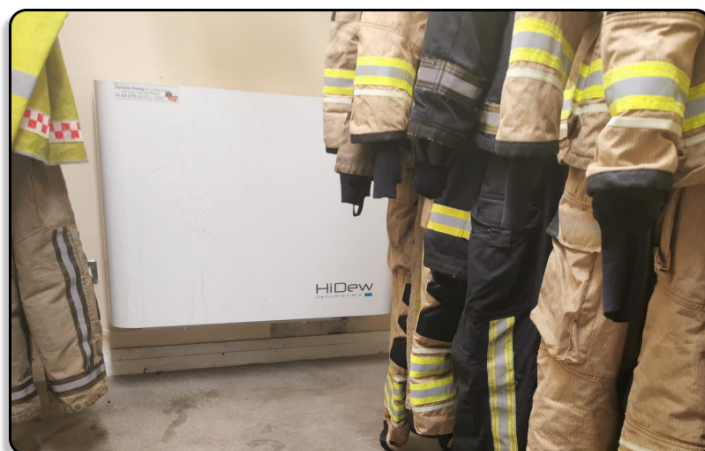
FIRE STATION DRYING ROOM WITH DDS DEHUMIDIFIER
