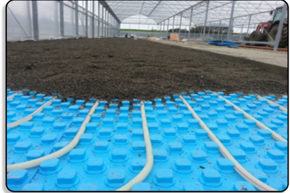
SWANTONS NURSERY, SKIBBEREEN AIR SOURCE (80kW) & UNDERFLOOR HEATING (ACCELERATES THE GROWTH PROCESS)
