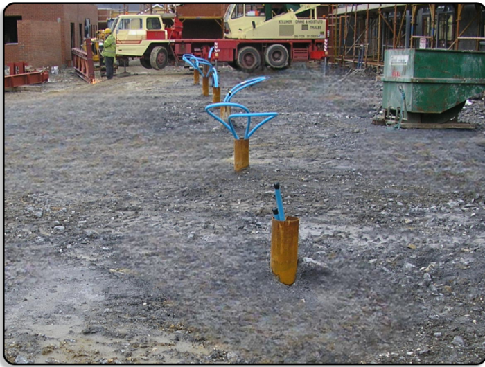
CLOSED VERTICAL BOREHOLE LOOP
