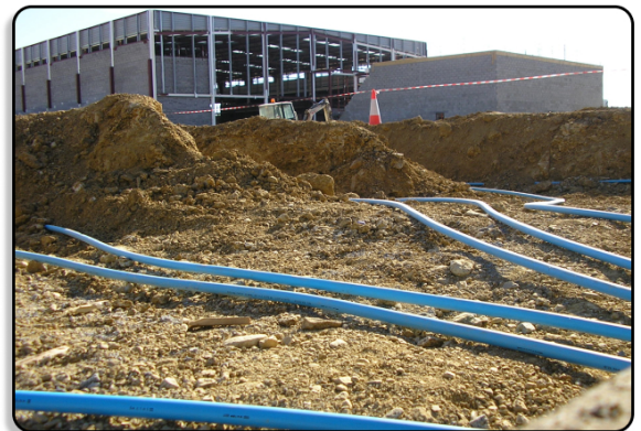
GAA SPORTS COMPLEX, MALLOW WATER TO WATER (68kW) CLOSED HORIZONTAL HEAT COLLECTOR
