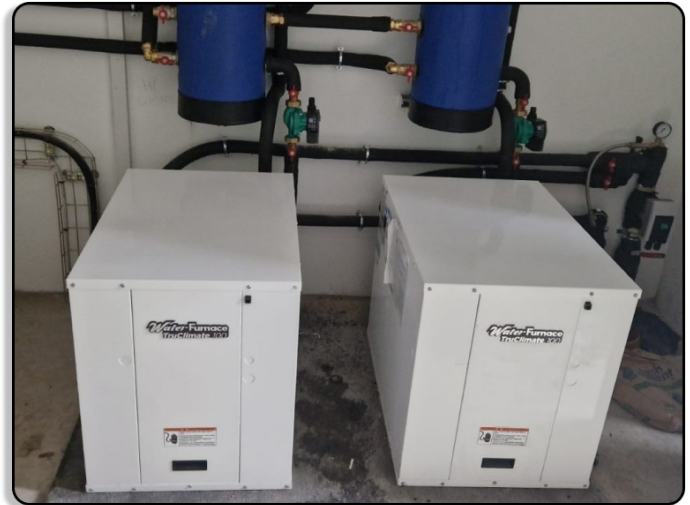
LARGE DOMESTIC, 17kW (ON HEAT ONLY) & 8kW ON HOT WATER + HEAT
