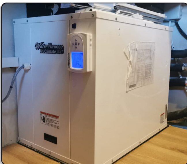
RESIDENTIAL, 12KW COOLING, X3 UNDERFLOOR ZONES & HOT WATER
