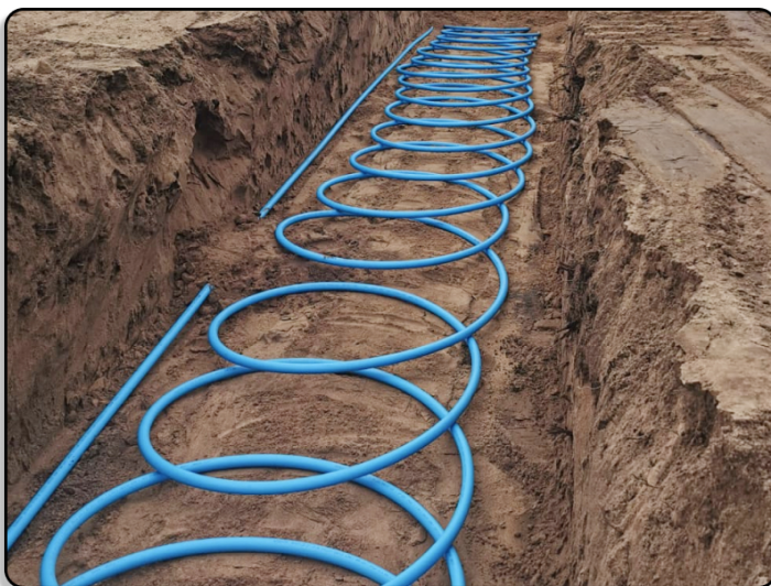
CLOSED HORIZONTAL LOOP
